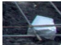
Concrete cover is the most important factor in protecting reinforcing steel from corrosion. The minimum concrete coverage for protection of reinforcement can be found in section 7.7 of ACI 318-08.
